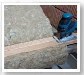
Furthermore, an **electric hedge trimmer** has proven to be a practical tool to cut insulation boards. With a 70 cm (length) long blade, a 60 cm board can be cut in one go. It is also helpful here to place a heavy wooden board on the insulation board and cut along the edge.
